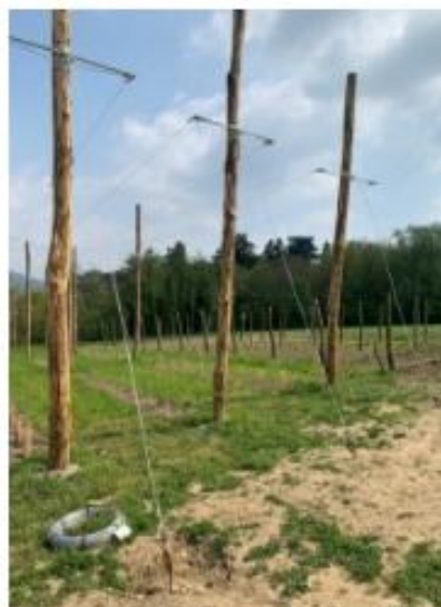
133 wire rope diam. 10 mm for anchoring
