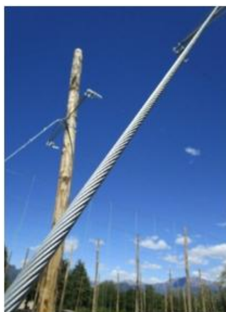
19 wire strand diam. 10 mm for supporting poles
