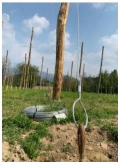
133 wire rope diam. 10 mm for anchoring
