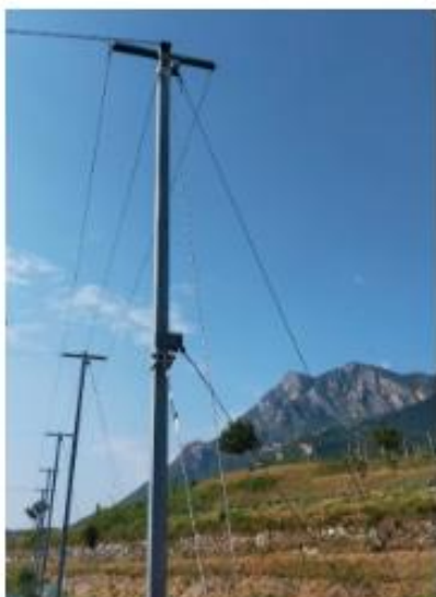
19 wire strand diam. 8 mm for anchoring
