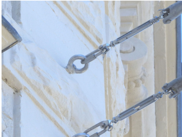
Anchoring of the supporting cable of subway, tramway and trolleybus catenary line (OHL).
