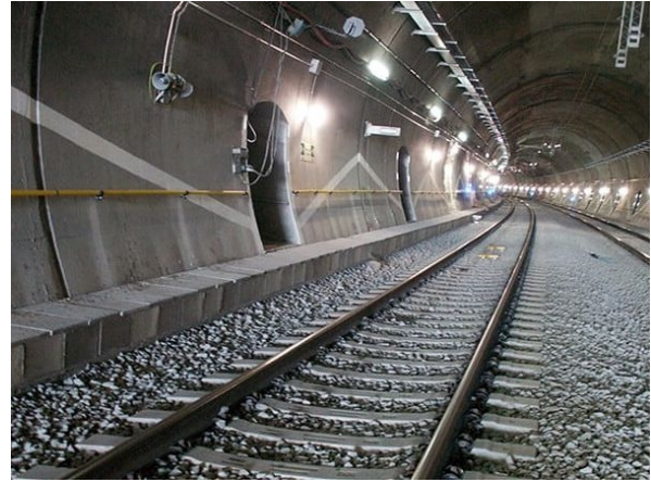
Anchoring of the supporting cable for installation of lighting, power and telecommunications lines in railway tunnels. Italian Railway Network (R.F.I): specification TT2482.
